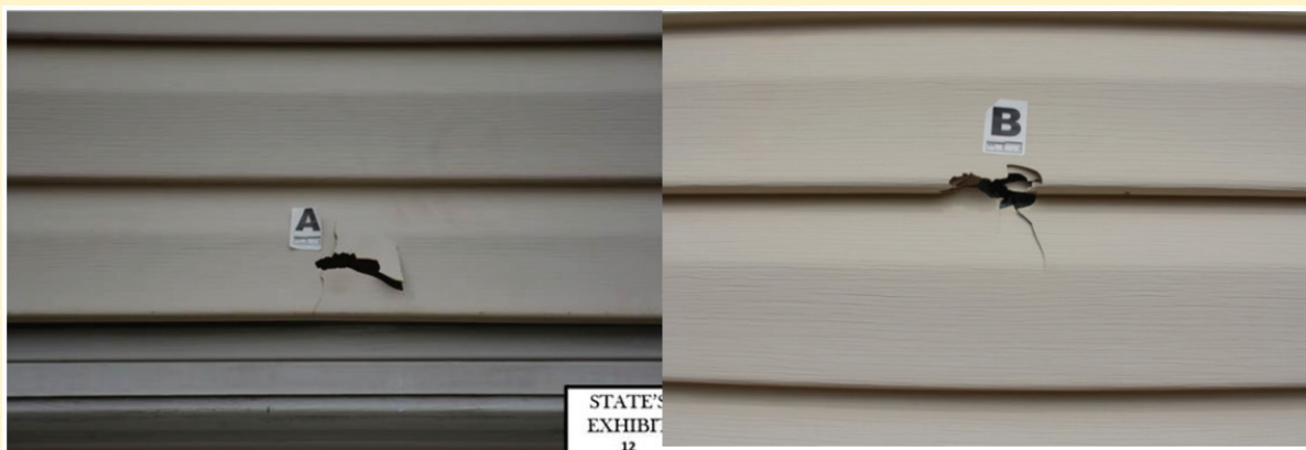
Figure A. Bullet holes repaired through the Goodwill Guardian Program
